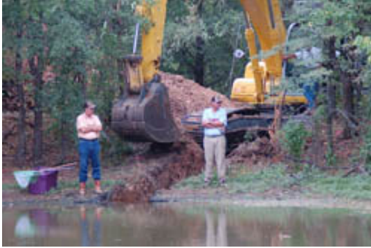
Employees of Mady Corporation standby as the draining trench is opened.
